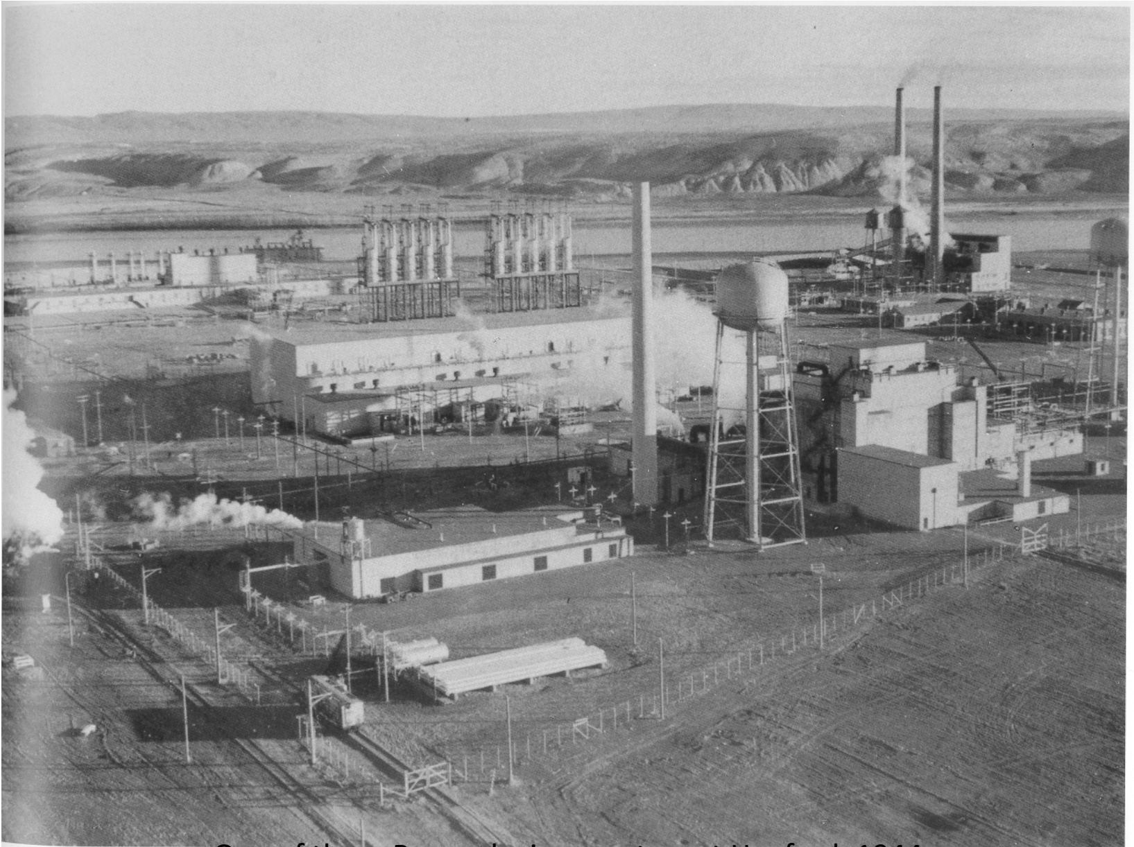
One of three Pu producing reactors at Hanford, 1944
